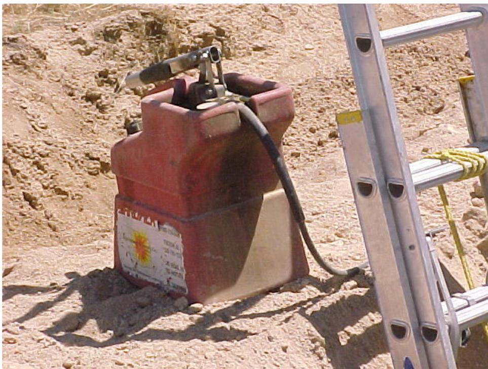
Notice the ladder is partially properly tied down. Three rungs out and tied but not staked.
