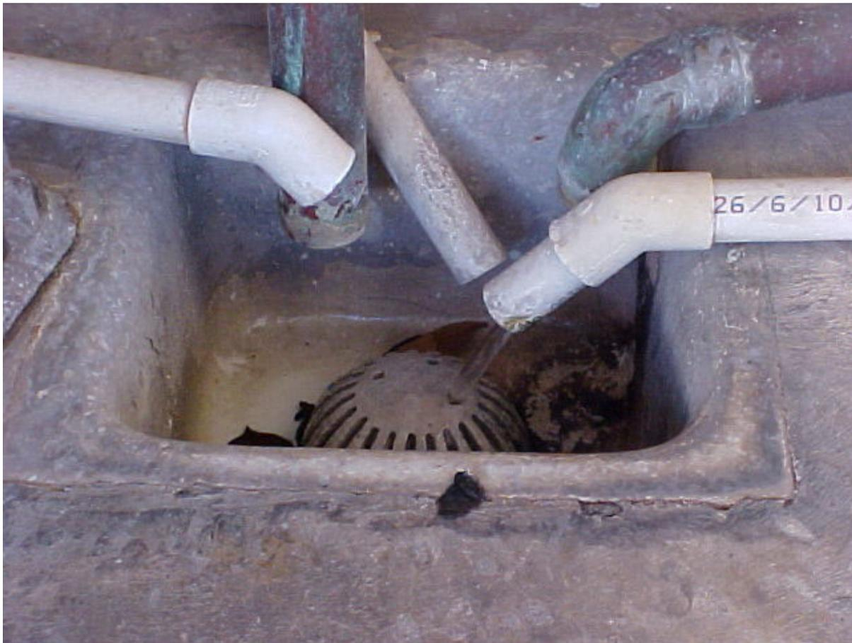
Which of these ice machine drains has an approved air gap? Here is a better question; would you use the ice from this ice machine? This is where all those stories about cockroaches and stomach flu originate.
