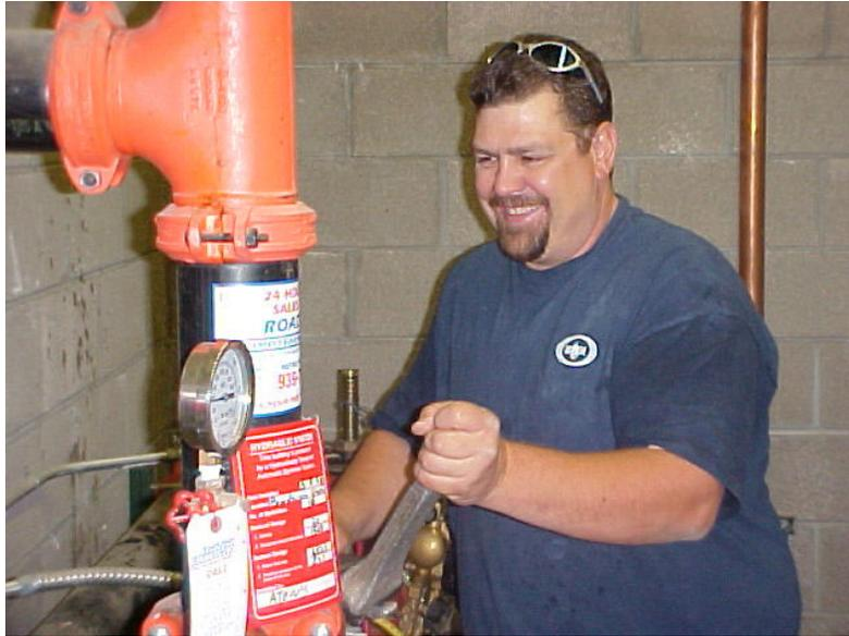
Top, a highly trained General Backflow Assembly Tester is working on a fireline assembly.
