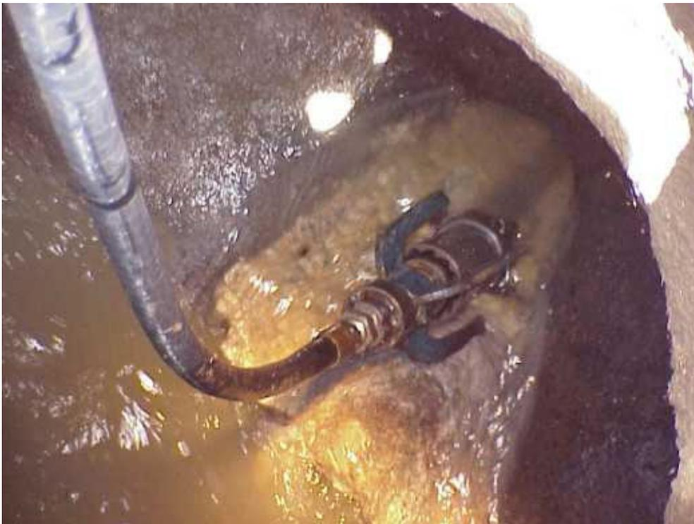
This is a sewer line that has a large amount of grease buildup that will be cut out. Grease gets into the sewer line by pouring grease left over from cooking, down the kitchen sink.
