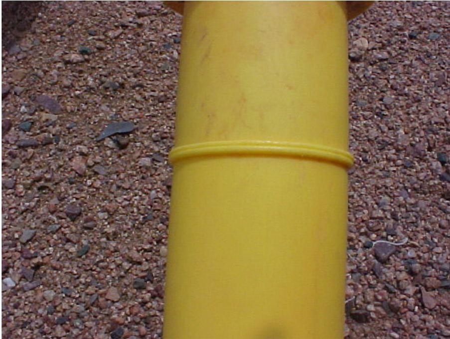
Fusion Butt Joint on plastic gas pipe.
