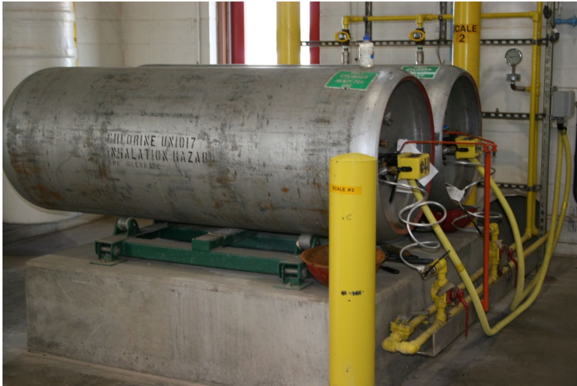
1-ton chlorine containers. Automatic shutoff device connected to the liquid side only. The top valve is used for the gas. Remember that containers lay on their sides and cylinders stand upright. Roller bearings should not be used to rotate the container because of the ease of rotation is too great.
