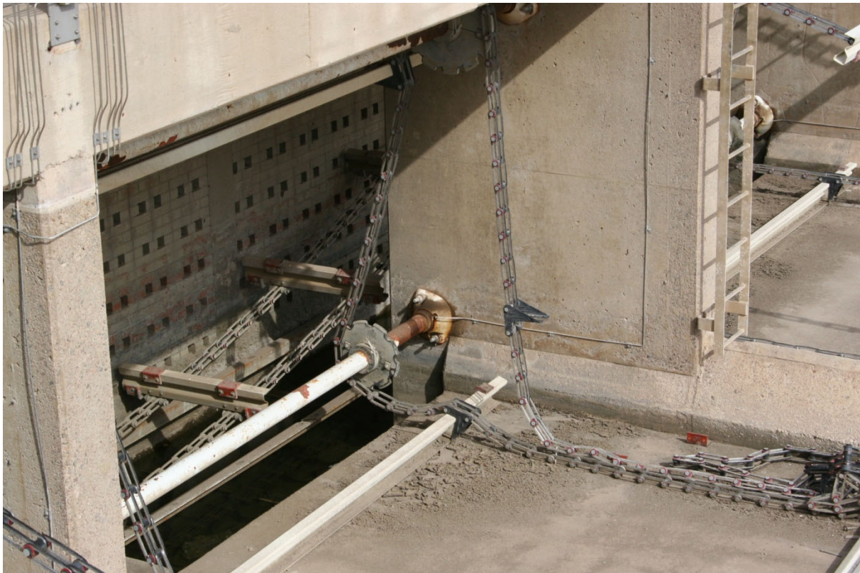
Rectangular basin flights and chains.
