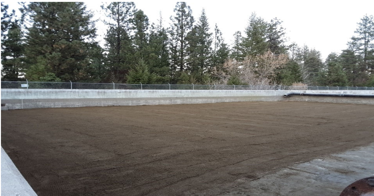
SLOW SAND FILTER These have become obsolete
