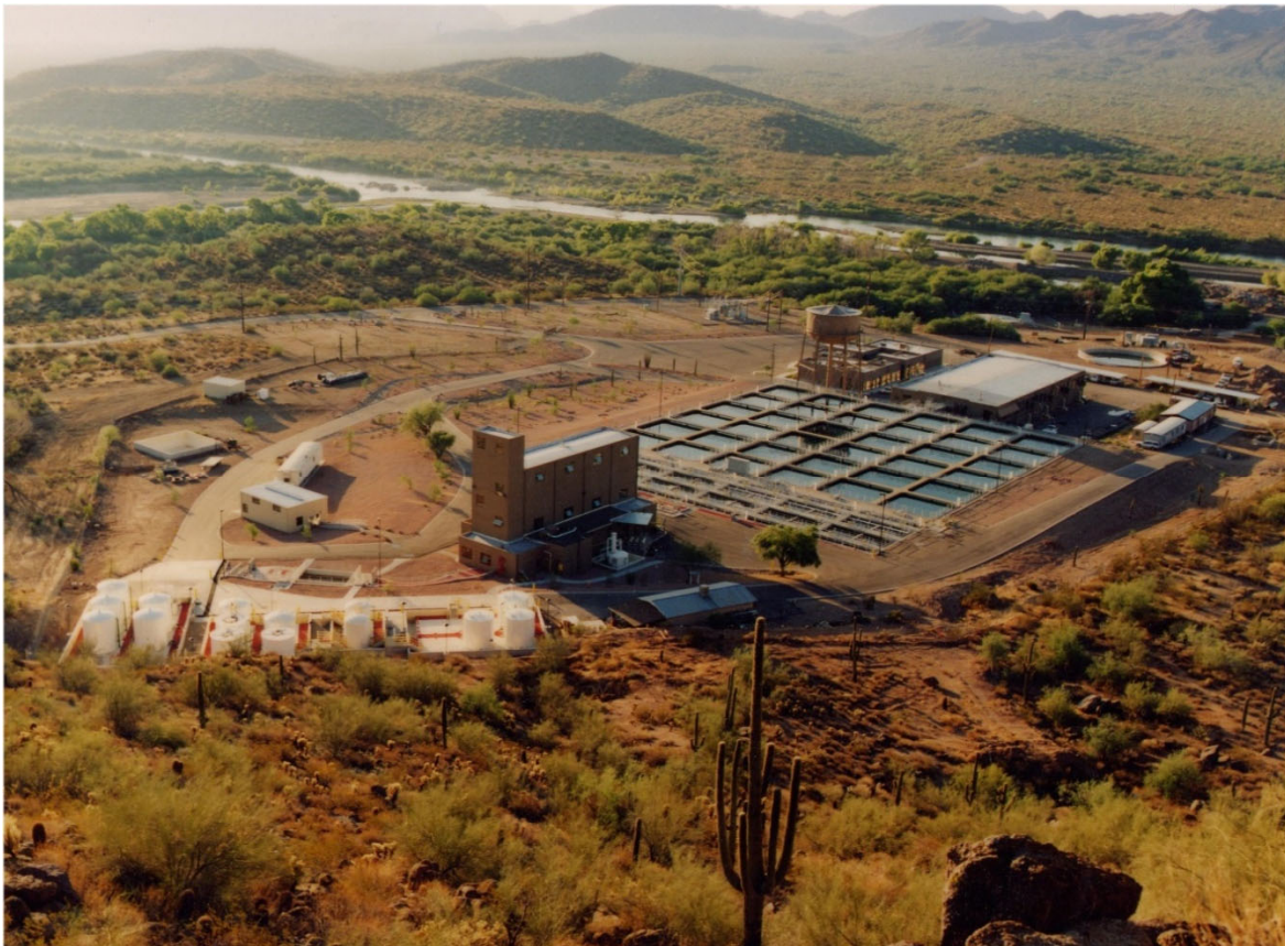
A surface water conventional treatment facility next to a river.
