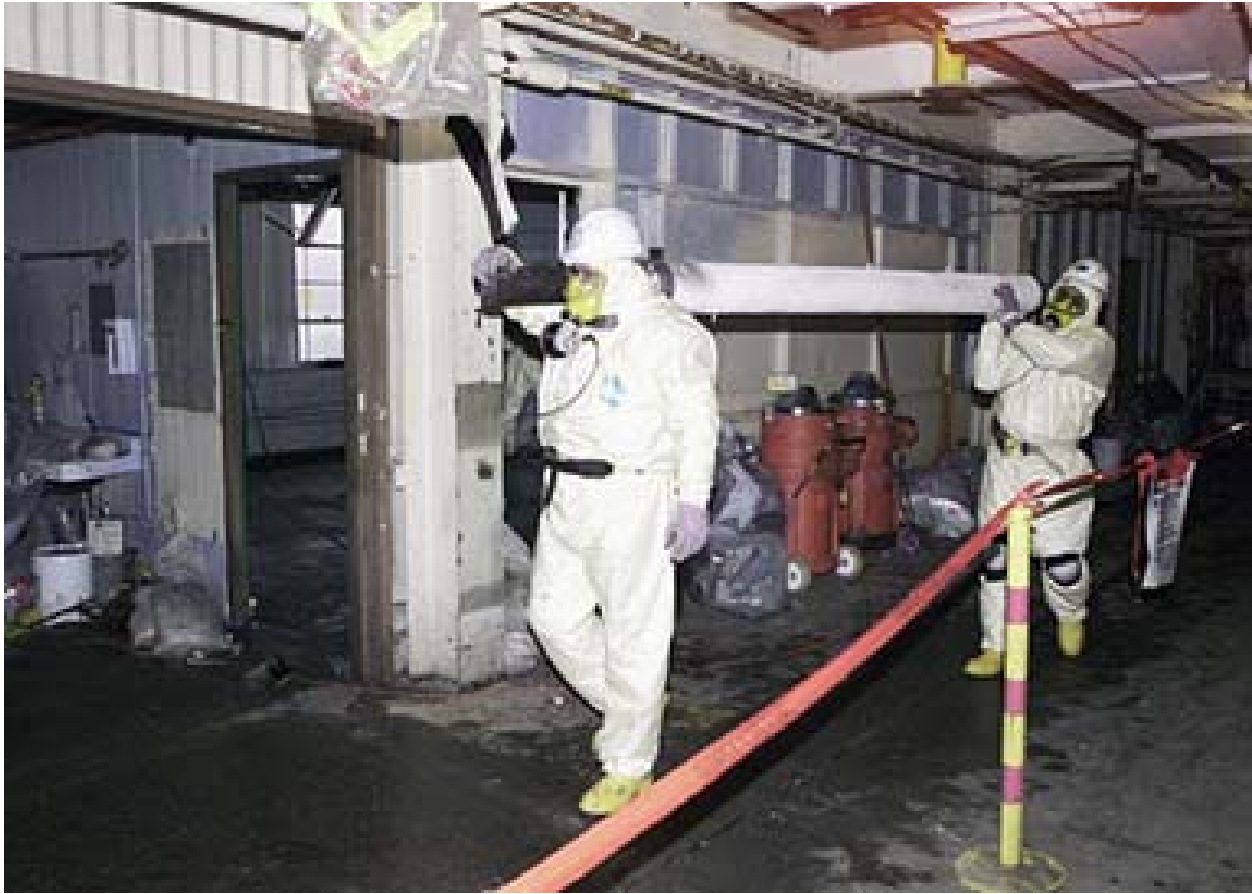
Workers removing Asbestos wrapped Pipe
