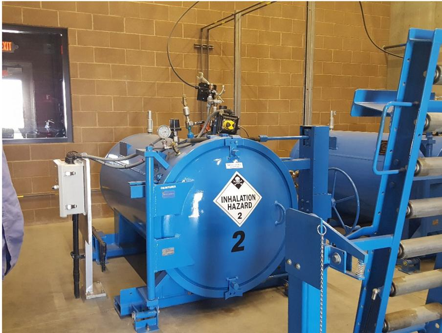
These photos are of high-pressure chlorine containment vessels into which a 1-Ton or 150-lb chlorine gas cylinder is processed. If the cylinder should leak, chlorine gas is contained within the vessel and processed at a normal rate. All of the chlorine gas is used and no hazardous waste is generated.
