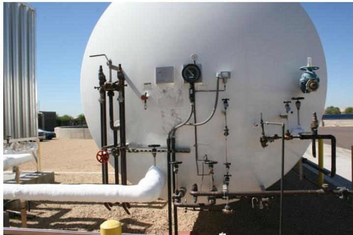
Oxygen tank is necessary to generate O<sub>3</sub>
