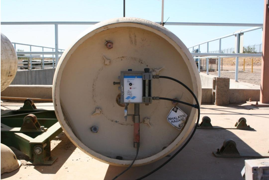
Hard to tell, but these are one-ton chlorine gas containers. Notice the five-gallon bucket of motor oil in the bottom photograph. Do you have an eye wash and emergency shower?
