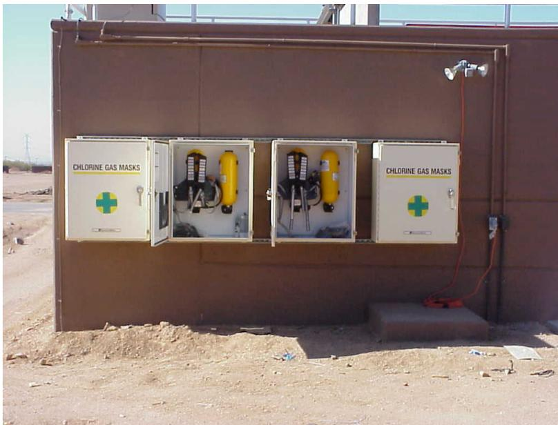
Staff shall be familiar with the locations of the chemical feed building as indicated by a posted site plan. Self-contained breathing apparatus (SCBA) and personal protective equipment should be facing the chemical feed building. Emergency repair kits “B” and “C” should be stored on site close to the chemical feed building.
