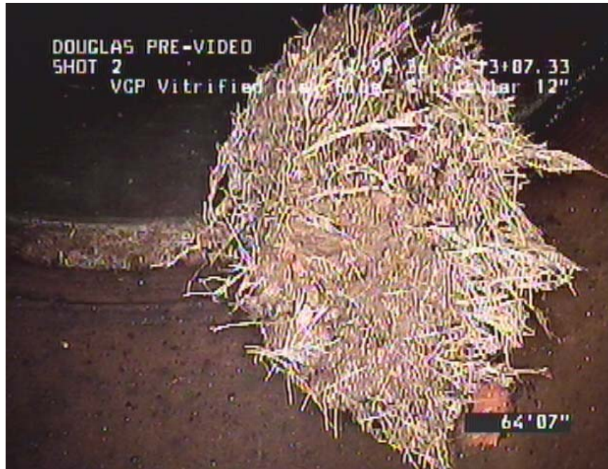
Root sewer blockage Photograph of sewers courtesy of Propipe.
