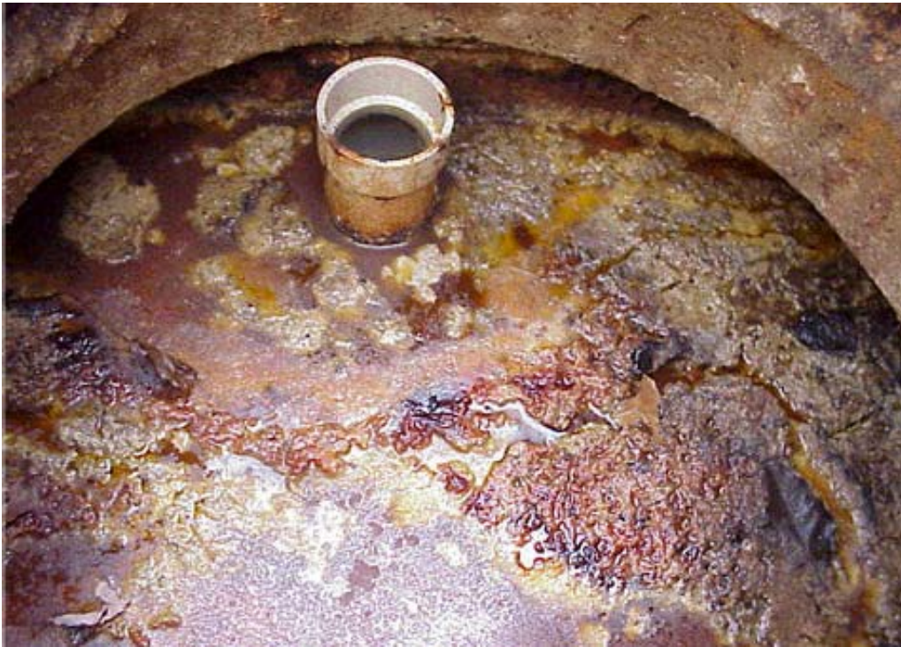
A grease interceptor used in a commercial food service operation.
