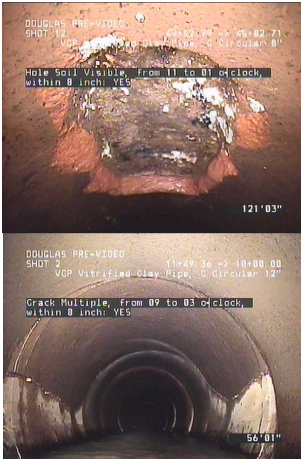
Examples of pipe corrosion. Photographs courtesy of Propipe.
