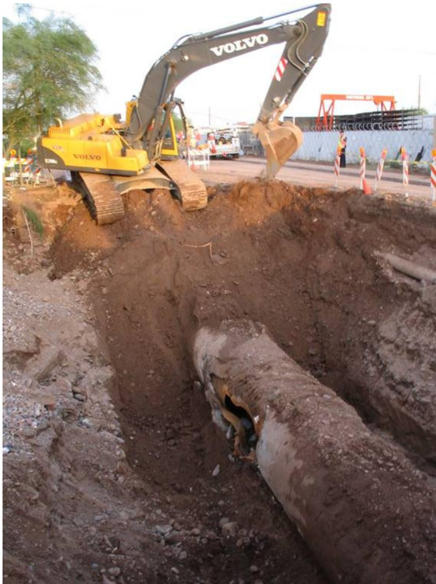
54-inch water main blow out. Are you prepared to handle this type of an emergency? Most water providers will have to contract this type of work out because they are not prepared.
