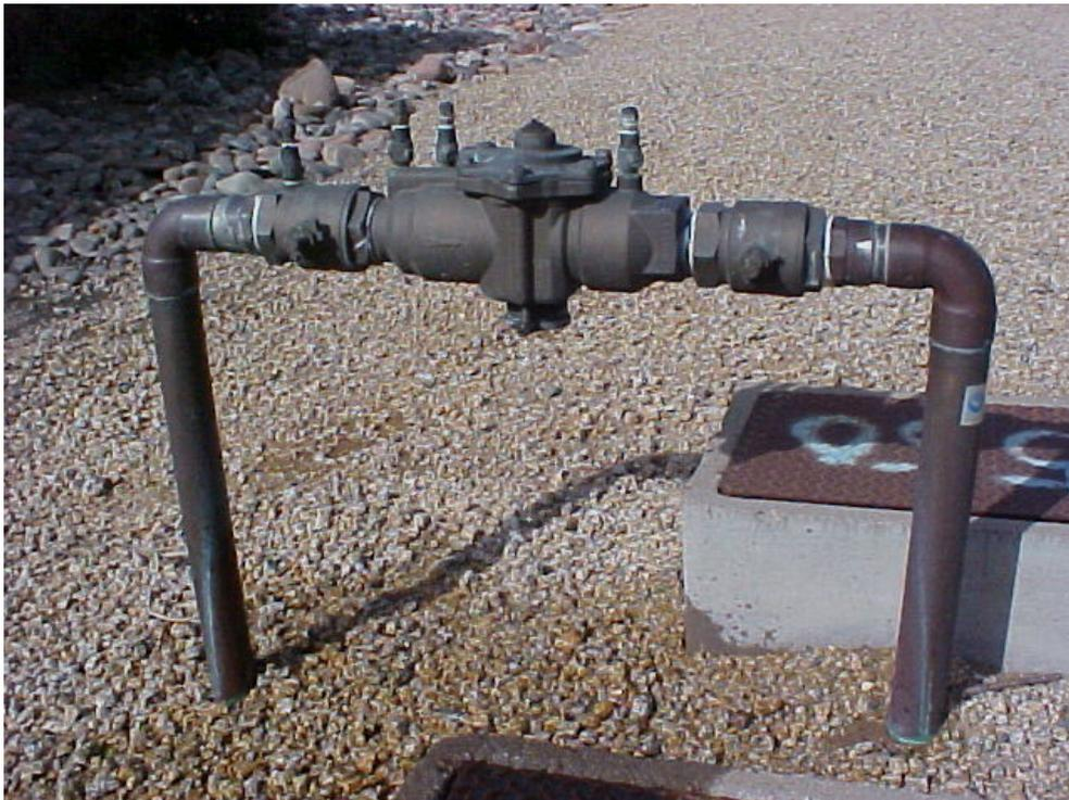
**Leaky RP**--have your assemblies tested annually or more often. Re-test after repairs and problems. A RP should not leak more than 1 or 2 minute—any more than that, there is a problem; a piece of debris or stuck check is causing the RP's hydraulic relief port to dump.
