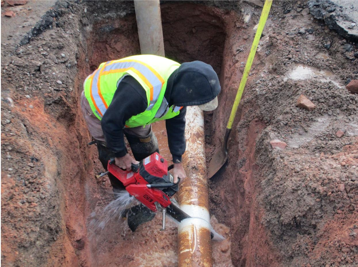
Cutting out a damaged water main section.
