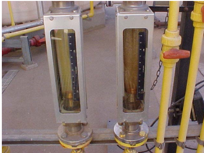
*Chlorine measurement devices or Rotameters
