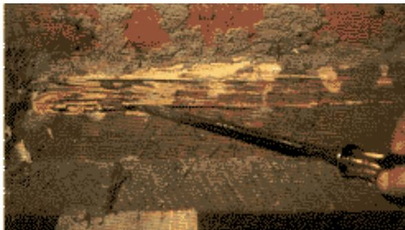
Using a screwdriver to examine termite damage, Subs will go with the grain.
