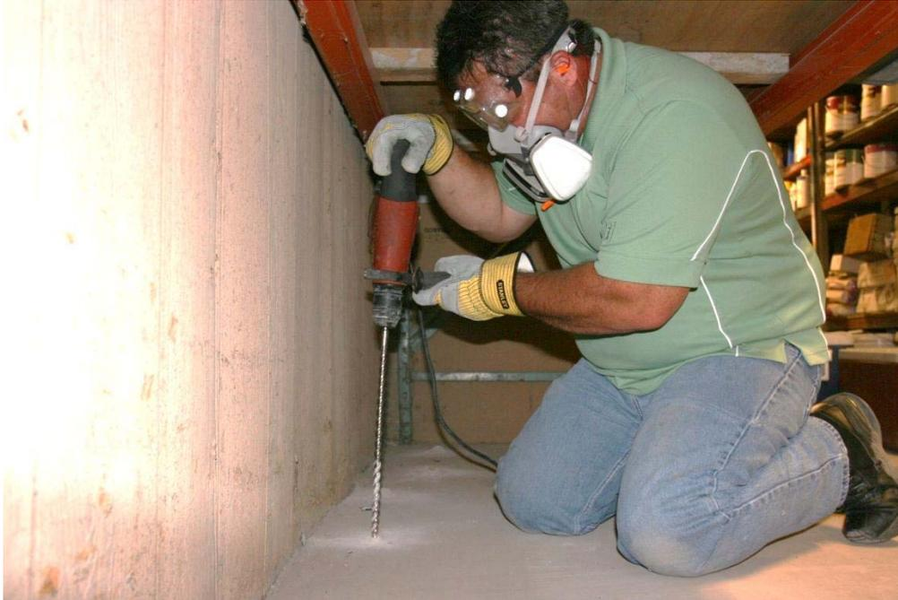
Drilling is hard work; there are days you might drill every day, it is best to work as a two-man team if you are doing termite treatments. Beware of hitting rebar and deep footers. After your first inspection, draw a detailed plan of action and map your treatment methods, this is required by law and good for your records and customers as well. Subs are easy to kill if you do a good treatment. It might take a month but they are walking dead.
