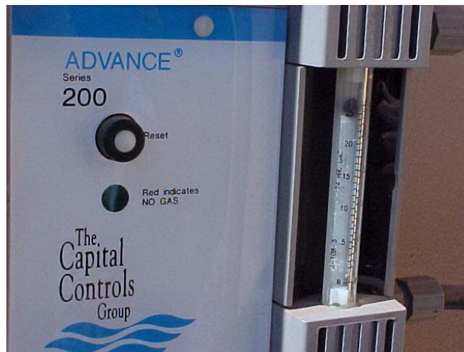
*Chlorine measurement devices or Rotameters
