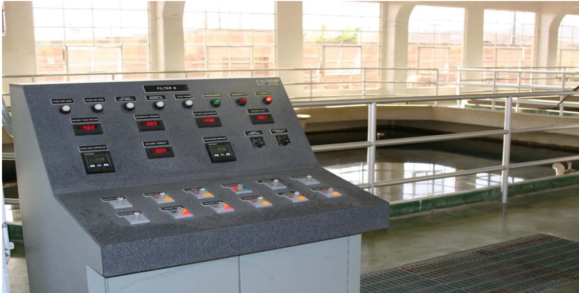
This is a filter control panel.
