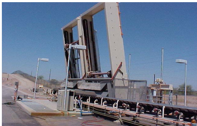
Mechanical bar screen
