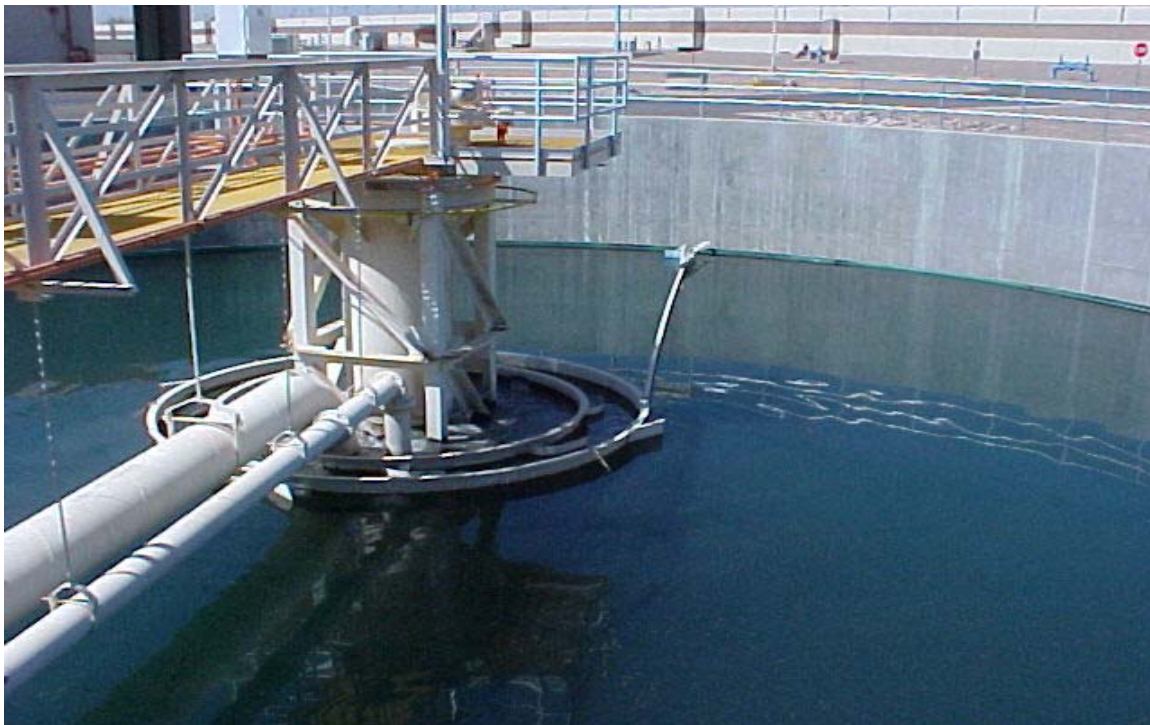
Circular clarifier and collector mechanism.
